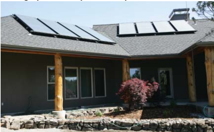
This Oregon home uses the power of the sun for water heating.
