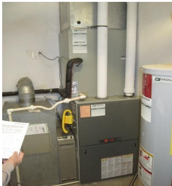
Figure 50: GF 1.0 Direct Vent Condensing Furnace
