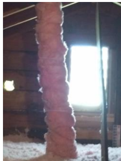
Figure 21: VE 1.2 Insulated Exhaust Vents to the Outside
