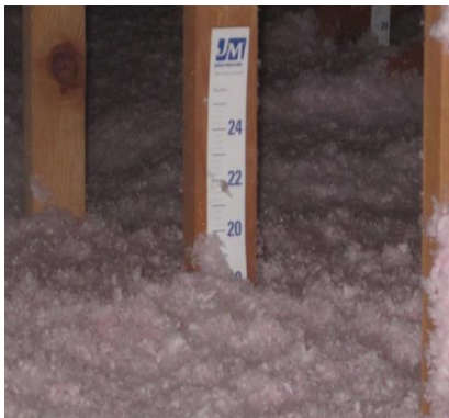
Figure 12: AT 2.2.1 Insulation Marker
