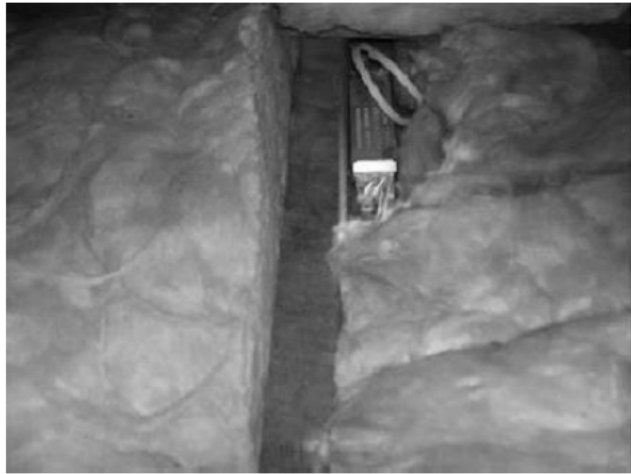
Figure 8: PR 1.4.2 Dams around light fixtures
