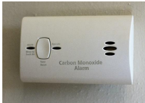
Figure 39: AS 1.0 Carbon Monoxide Detector
