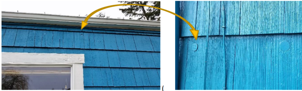
Figure 37: WA 1.1 Exterior Wall Plugs
