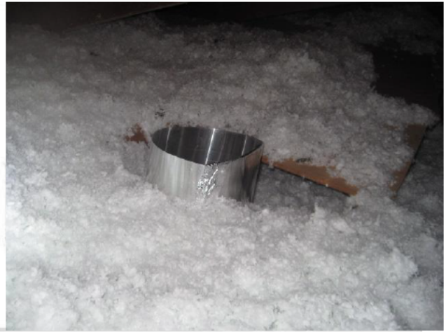
Figure 8: PR 1.4.2 Dams around light fixtures
