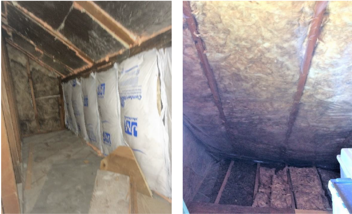
Figure 16: AT 2.3 Kneewall insulation
