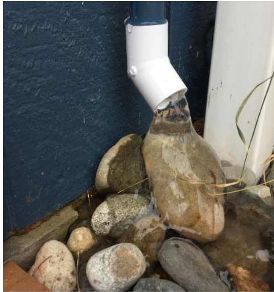
Figure 51: GF 1.2 Ice Dam at Condensate Termination
