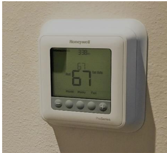
Figure 56: PT 1.1 Honeywell Programmable Thermostat
