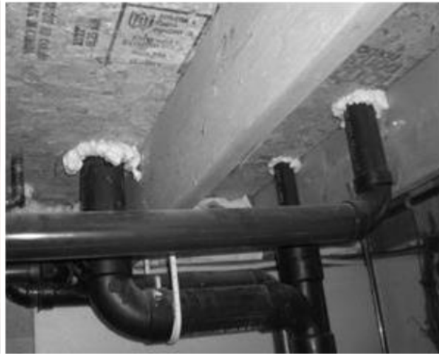
Figure 26: FL 1.3 Floor Penetrations
