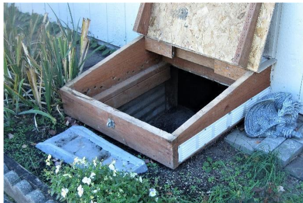
Figure 34: FL 2.5 Horizontal Crawlspace Access
