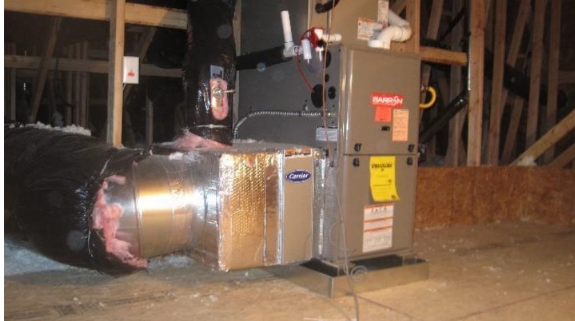
Figure 46: DU 1.3 Duct Insulation and Duct Seal
