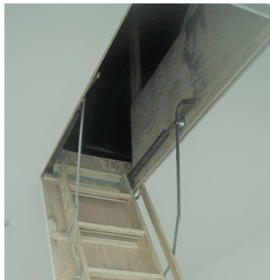
Figure 11: AT 1.1.2 Attic Access w/ Dam
