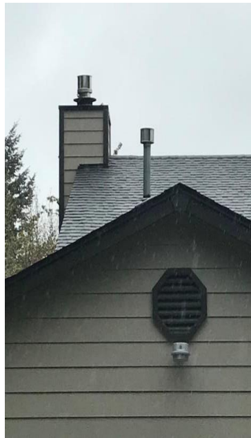
Figure 23: VE 1.5 Exhaust Vents
