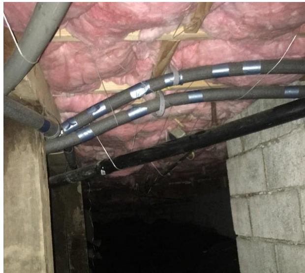
Figure 32: FL 2.3 Water Pipe Wrap
