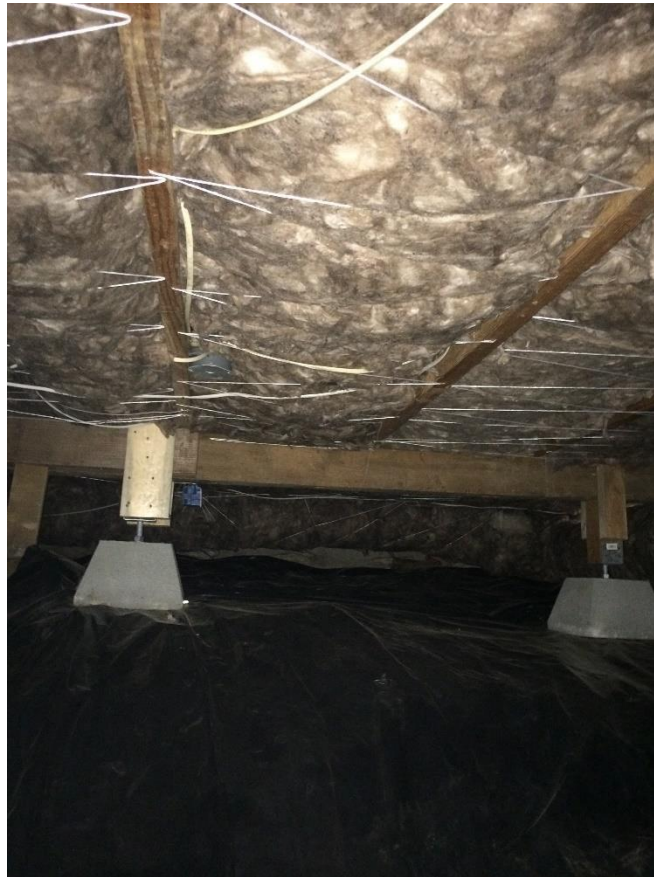
Figure 24: FL 1.0 Supported crawlspace insulation and groundcover
