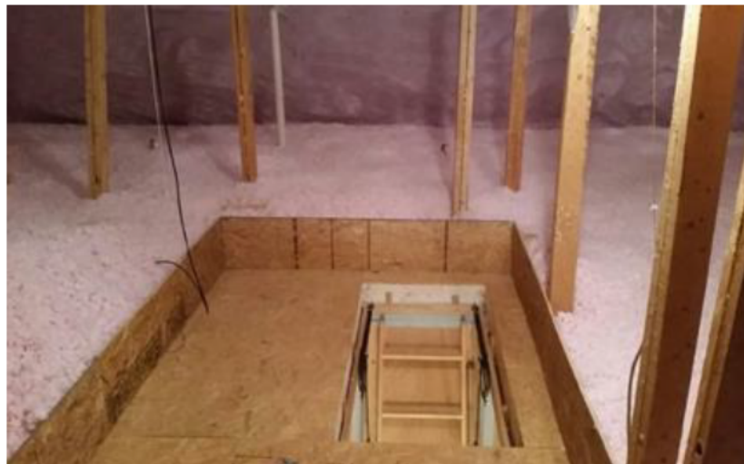
Figure 5: PR 1.3.2 Attic Access damming
