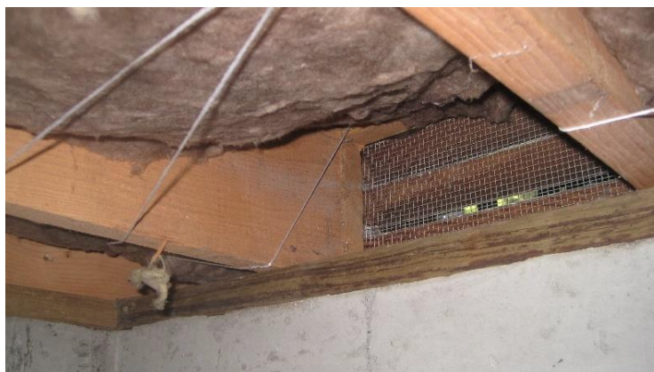
Figure 22: VE 1.5 Crawlspace Ventilation
