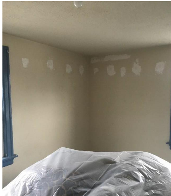
Figure 38: WA 1.4 Interior blown insulation
