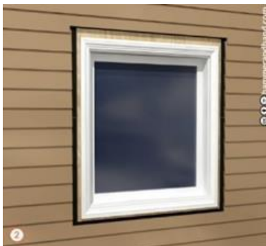
WI 1.2 – Carefully remove existing trim and try to salvage for use after new window is installed.
