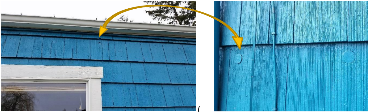
Figure 37: WA 1.1 Exterior Wall Plugs
