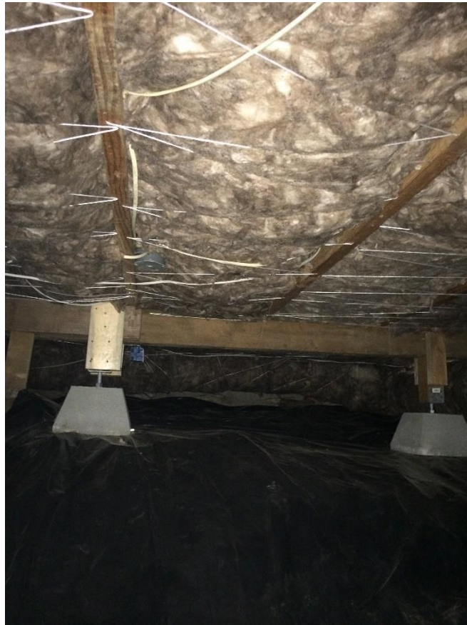
Figure 24: FL 1.0 Supported crawlspace insulation and groundcover
