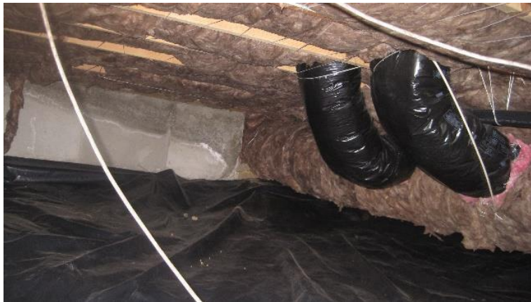
Figure 48: DU 1.4.2 Insulation Covered
