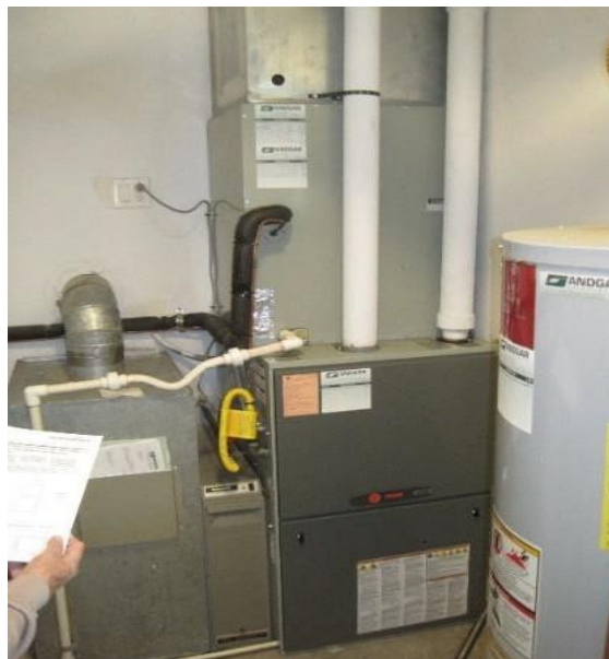
Figure 50: GF 1.0 Direct Vent Condensing Furnace
