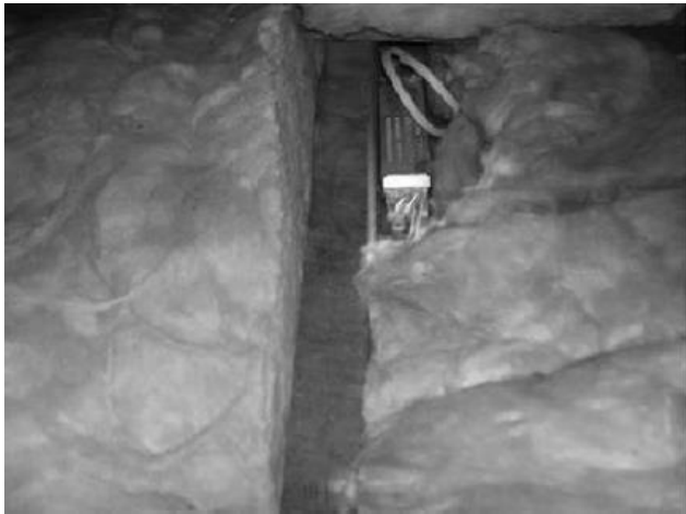
Figure 8: PR 1.4.2 Dams around light fixtures
