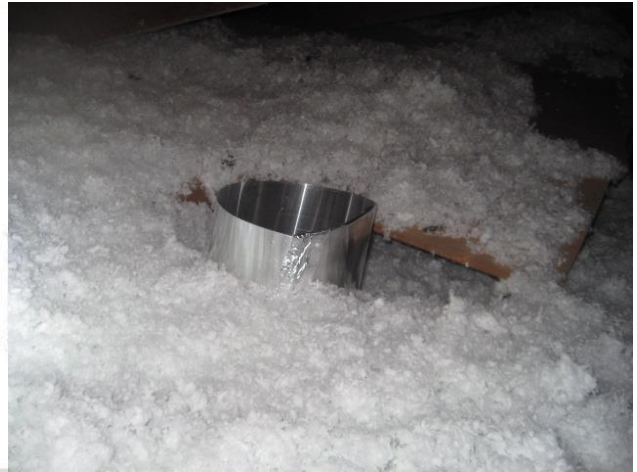
Figure 8: PR 1.4.2 Dams around light fixtures
