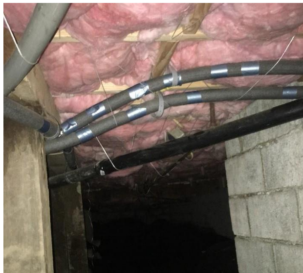
Figure 32: FL 2.3 Water Pipe Wrap
