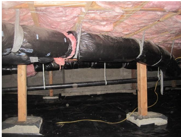
Figure 42: DU 1.6 Correctly supported ducts
