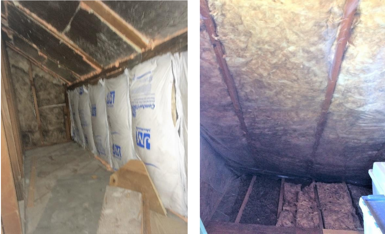
Figure 16: AT 2.3 Kneewall insulation
