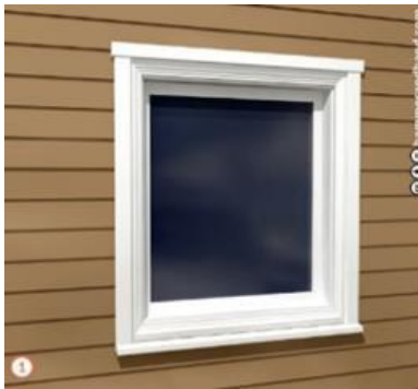
WI 1.1 – Existing conditions to be retrofitted.
