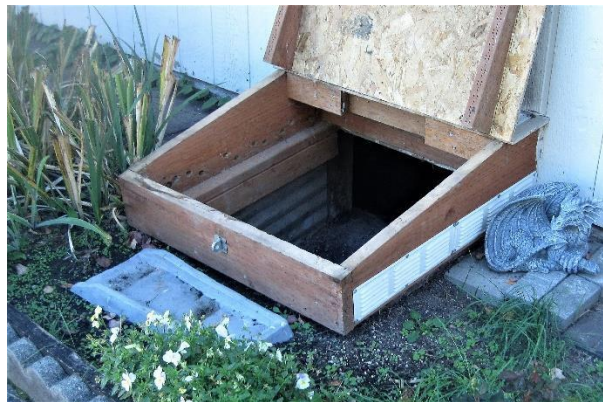
Figure 34: FL 2.5 Horizontal Crawlspace Access
